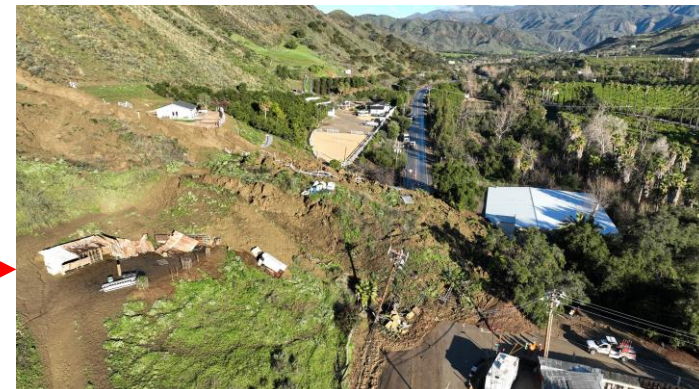
Credit: Caltrans District 7
