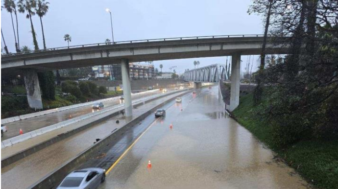
Credit: Caltrans District 7
