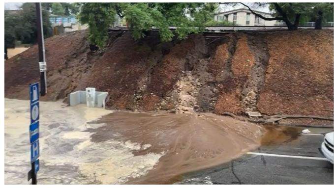
A hillslope failure due to heavy rains combined with floodwaters to force roadway closures in Santa
