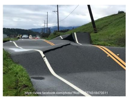
Severe damage was caused to a roadway in Marin County due to a hill slope failure, resulting in buckling of the road Olompali State Historic State Park
