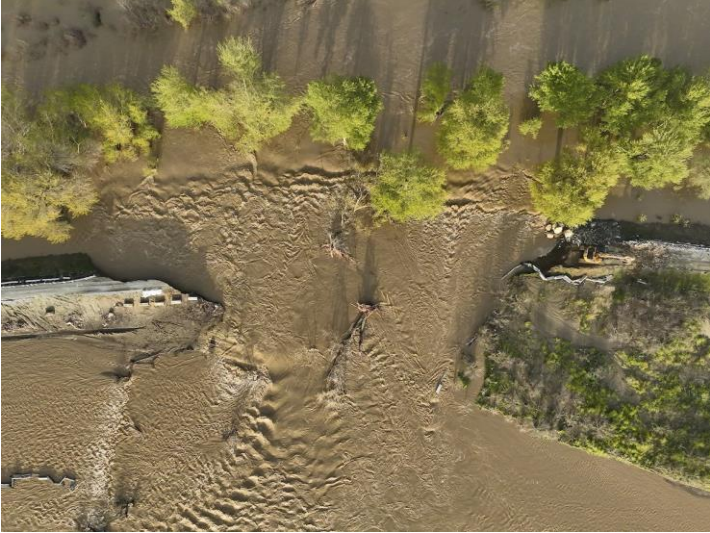
Levee break on the Pajaro River California DWR Twitter
