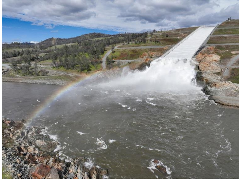
Lake Oroville Spillway www.resources.ca.gov
