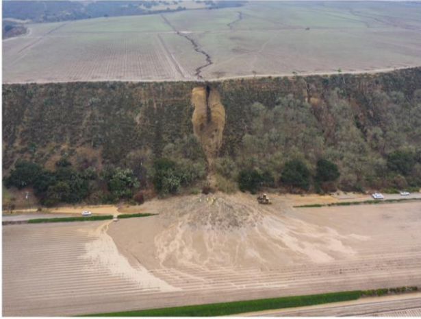
Mudslide along River Road near Salinas, CA
