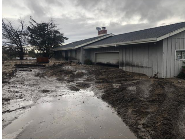
Home Damaged by Mudslide near River Road
